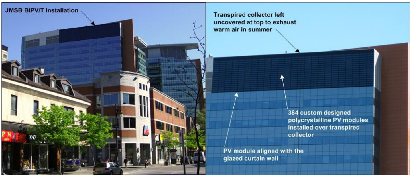
Street and Detailed View and of John Molsen School of Business Solar Wall, Concordia University, Canada.
